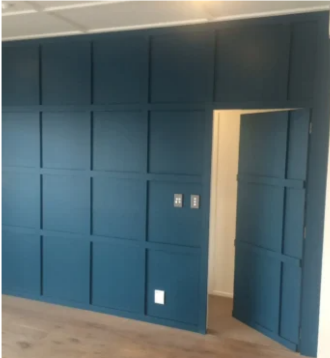
Paneled Wall W/ Hidden Door for Closet Storage Paint Trim Color
